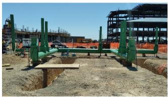
More than 6,000 feet of PP-RCT piping was installed at the United States Air Force's Joint Base San Antonio-Lackland, Texas for hot and cold potable water, non-potable HVAC heating and chilled water, plus condenser water. The pipe was selected for its greater pressure capabilities at higher temperatures than conventional PP materials.
